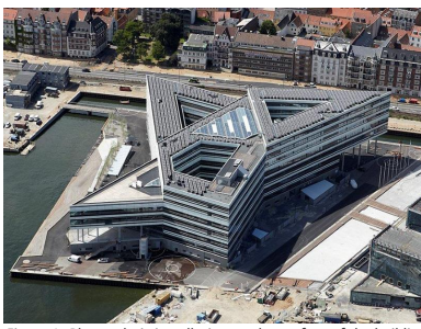
Figure 1: Photovoltaic installation on the rooftop of the building that will be used in this project.
